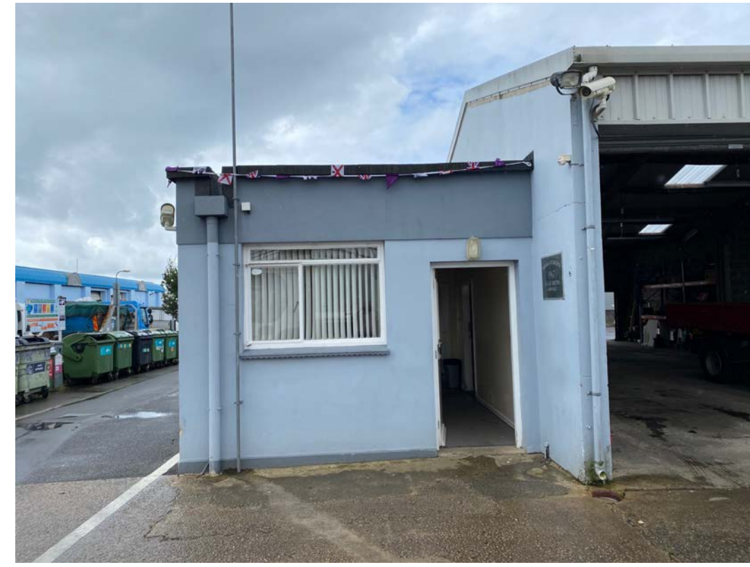
photo - north east elevation
