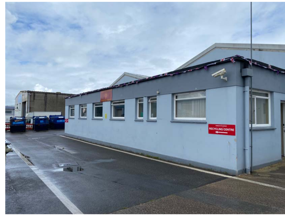
photo - south east elevation
