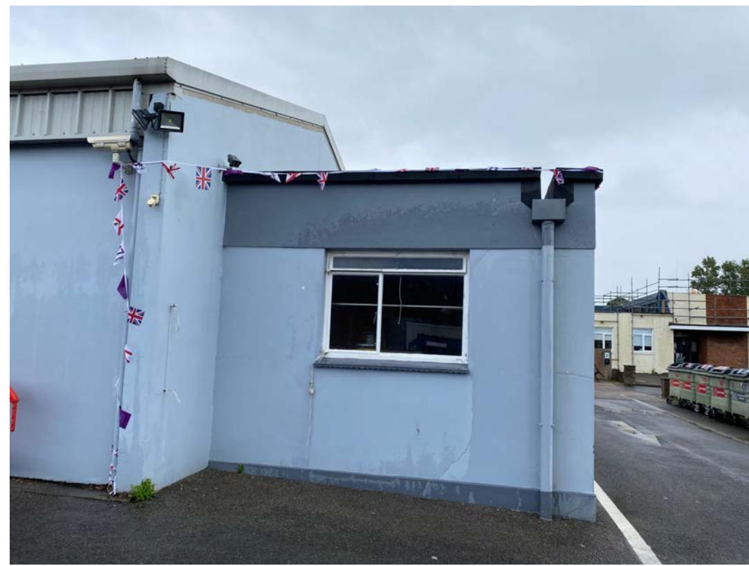
photo - south west elevation
